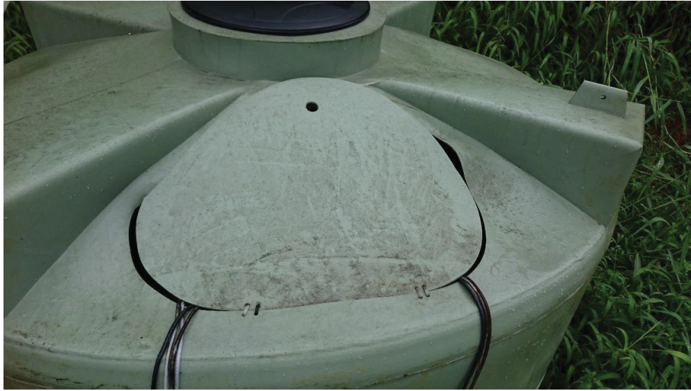
Figure 7. Door to access the tank with cable tie hinges
