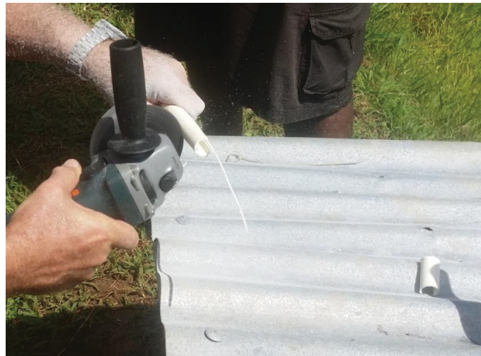
Figure 12. Picture showing the cutting of clips from 25mm PVC
