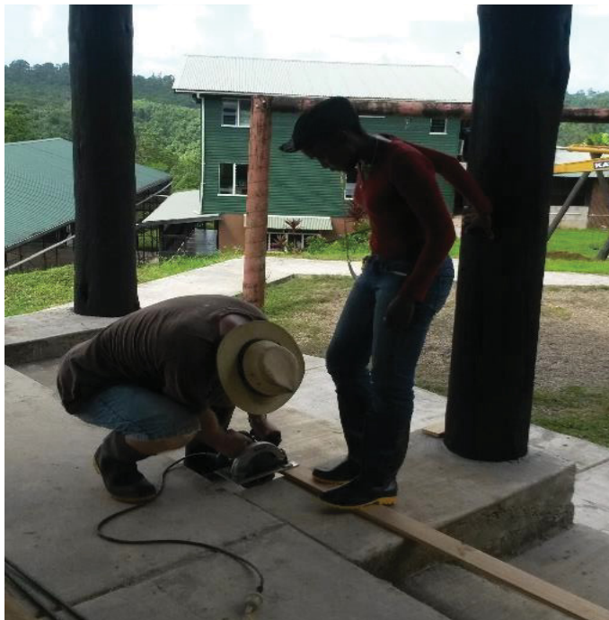
Figure 5. Timber being cut to requisite lengths using power saw
