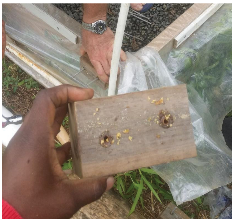
Figure 13. Blocks of wood to be used to mount the lock channel
