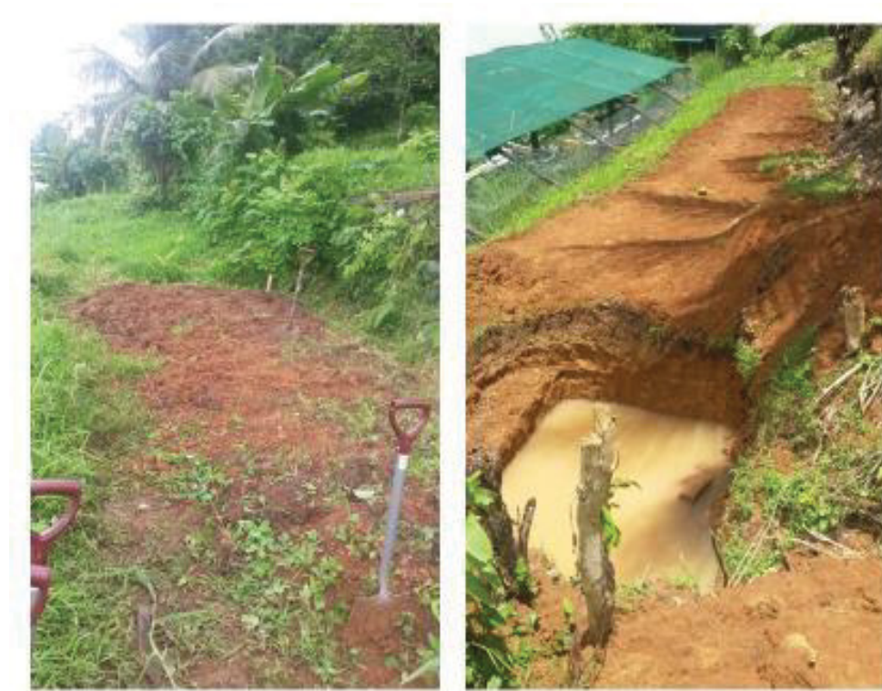
Figure 4. Preparation of area for aquaponics system by digging a hole for the water tank and levelling the grow bed area.
