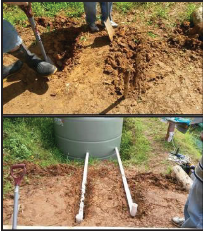
Figure 8. Digging of trenches for drain pipes and subsequent installation of the drain pipes
