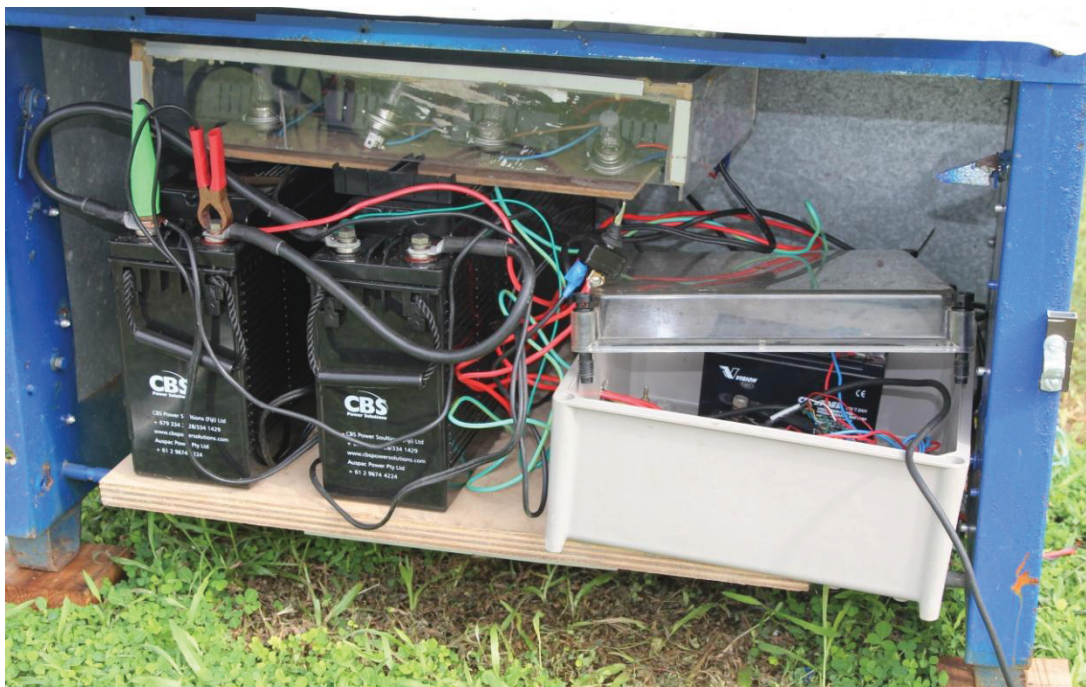
Fig. 6.5 Monitoring station consisting of battery bank, electrical loading and data logging equipment
