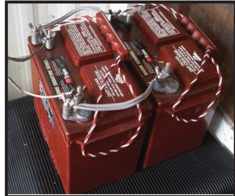
Figure 2.8 Trojan batteries (load bank)
